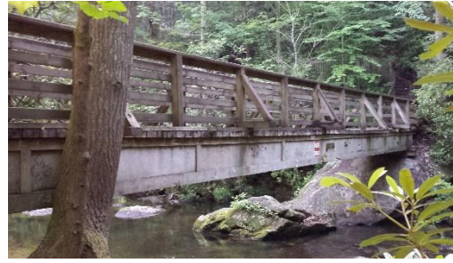
Example of Bridge – SMSP
